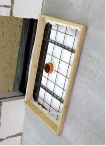
Concrete deck moulded around the recess
