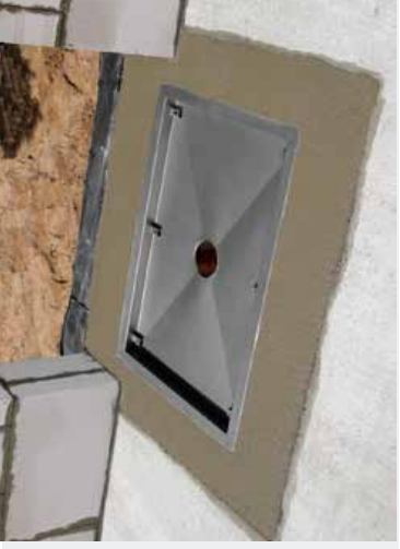
When the MatLine unit is positioned correctly, mould concrete around it
