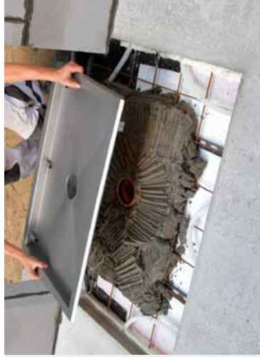
Fit the MatLine system onto the sewer pipe and press into the concrete
