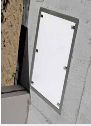
Place the protective foam block (supplied) in the basin until installation is complete
