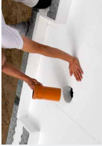
Insert the shortened pipe into the P-trap
