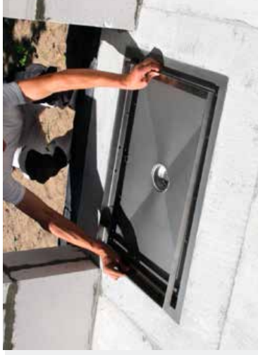
Fit the MatLine frame just before tiling
