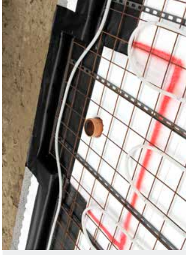
Lay iron mesh and underfloor heating pipes
