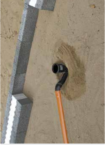
110 mm P-trap in position in the ground
