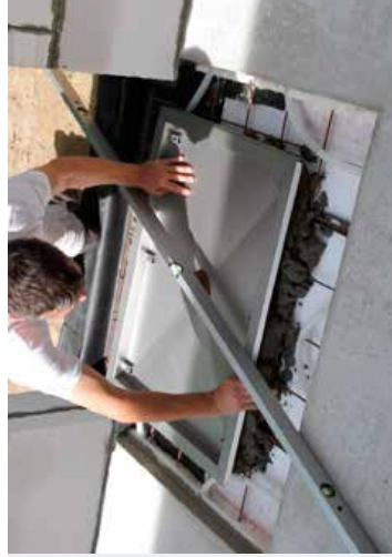
The top of the unit should be flush with the moulded concrete deck
